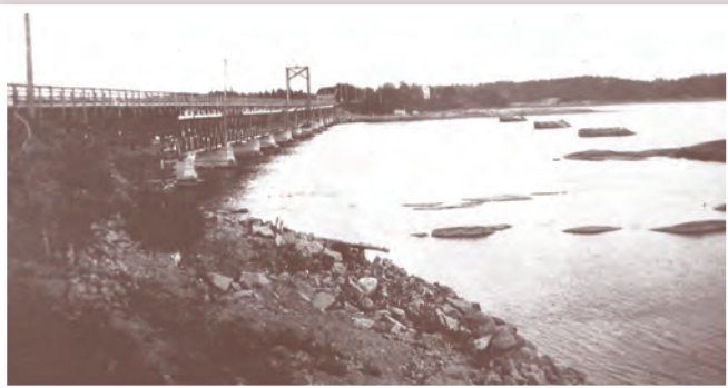
The first wooden Winnipeg River Bridge completed in 1908 had a swing span that opened to allow boats and barges through. Prior to the water raising in 1954, rock outcrops and currents near the bridge made navigation difficult. The west end collapsed under a City of Winnipeg Locomotive in 1914. This troublesome structure was finally replaced in 1931 by a new steel bridge by McCaw and MacDonald.
